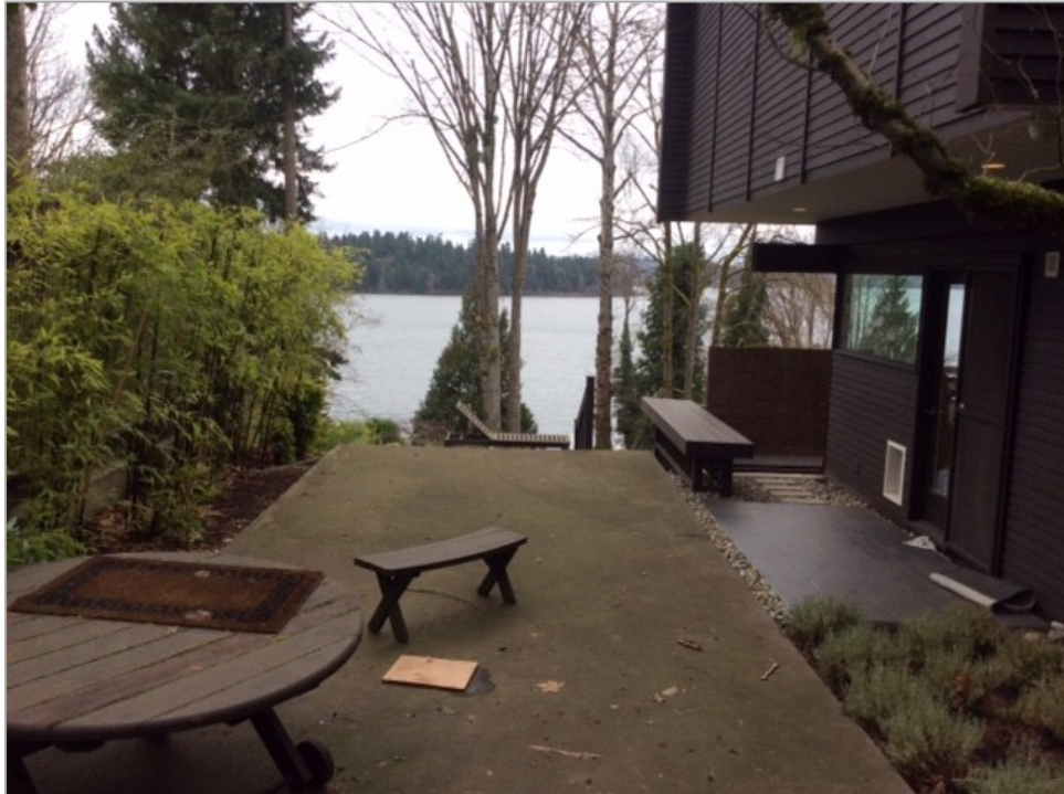
Photo 12a — Paved patio at 8101 SE 48 th Street, which contributes runoff into subject stormwater pipe.
