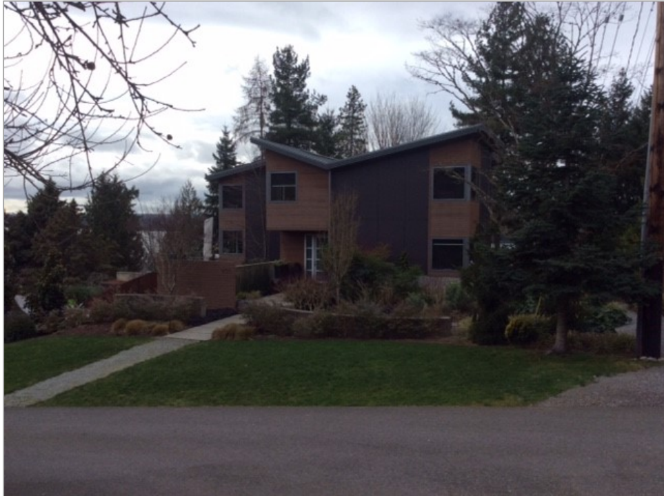
Photo 5 — New construction at 8105 SE 48 th Street, which contributes runoff into subject stormwater pipe. See photo for rear/side yard and driveway.
