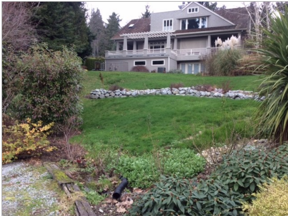
Photo 2 — 4803 W Mercer Way backyard. Note pipe, which discharges runoff onto parking pad and contributes runoff directly down drive to 8101 to subject stormwater pipe.
