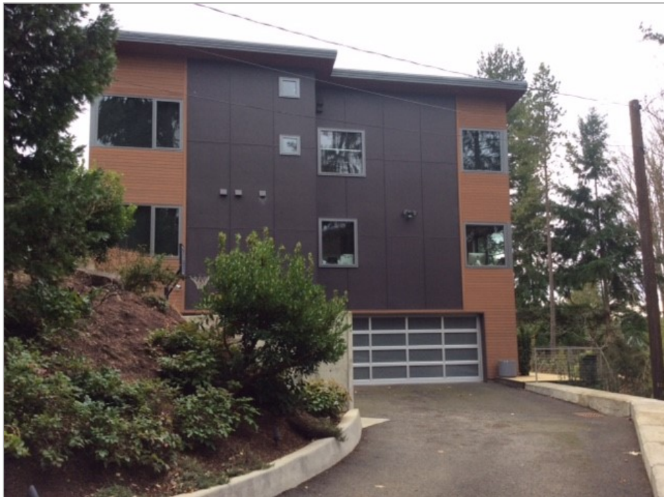
Photo 14 — New construction at 8105 SE 48 th Street, which contributes runoff into subject stormwater pipe. Note new catch basin in driveway (See Photo 9b).
