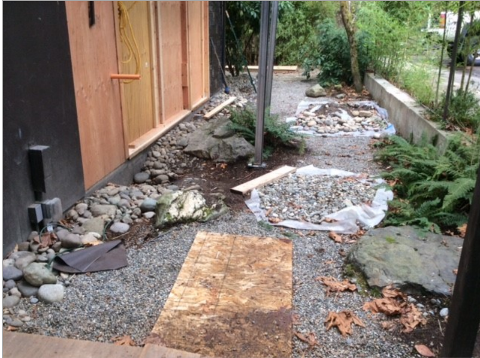
Photo 13 — New gravel and landscape area on east side of 8101 SE 48 th Street, looking north. Area captures runoff from paved driveway (See Photos 10 and 11).
