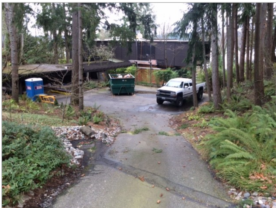
Photo 9b — Paved driveway of 8101 SE 48 th Street with new catch basin, which contribute runoff into subject stormwater pipe.
