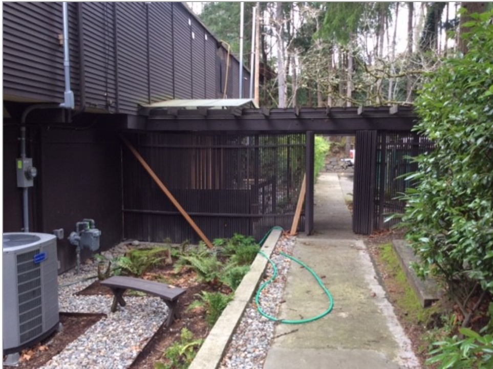
Photo 12b — Paved walkway at 8101 SE 48 th Street, which contributes runoff into subject stormwater pipe.
